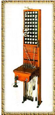
1890 Hasler LB Drop Switchboard
